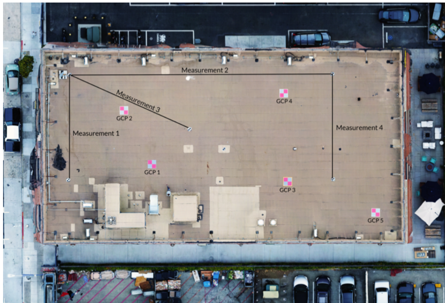
Figure 5. Aerial View of Ground Control System
